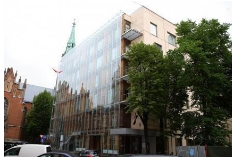
A-Class office building 'Baznicas 20/22'
