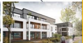
2 Apartment Houses (29 apartments) Construction Q2.2018.-Q2.2019.
