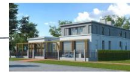
Villa Helena Construction started—till Q2.2018.
