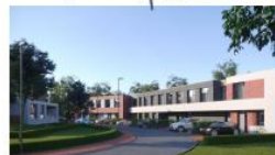
Row House (9 sections) Construction Q3.2018.-Q3.2019.
