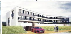
Apartment House (27 apartments) Construction Q3.2018.-Q3.2019.
