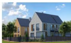
Twin Villa Magnolia Construction Q4.2017.- Q4.2018.
