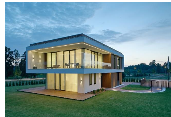
/Villa Corylus – construction finished/
