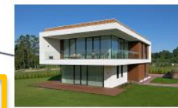
Villa Corylus Construction finished
