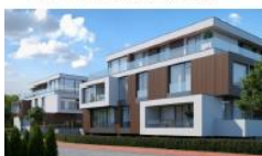
Apartment House (22 apartments) Construction Q4.2017 - Q4.2018
