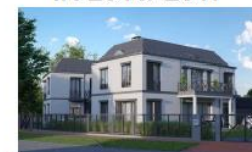
Twin Villa Camellia Construction started—till Q1.2018
