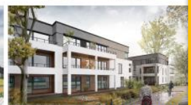
2 Apartment Houses (29 apartments) Construction Q2.2018 - Q2.2019
