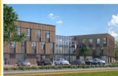
Public Building with Offices Construction Q2.2018 - Q2.2019
